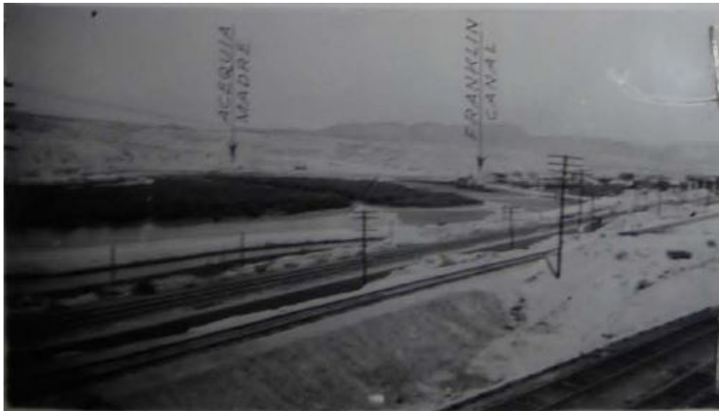
Rio Grande, Acequia Madre, and Franklin Canal below the International Dam with arrows indicating the locations of headgates of the two canals. Records of the Bureau of Reclamation. Engineering and Research Center Project Reports, 1910-1955, Box 722, Mexican Canal Diversions in the Vicinity of El Paso. U.S. National Archives, Denver.
