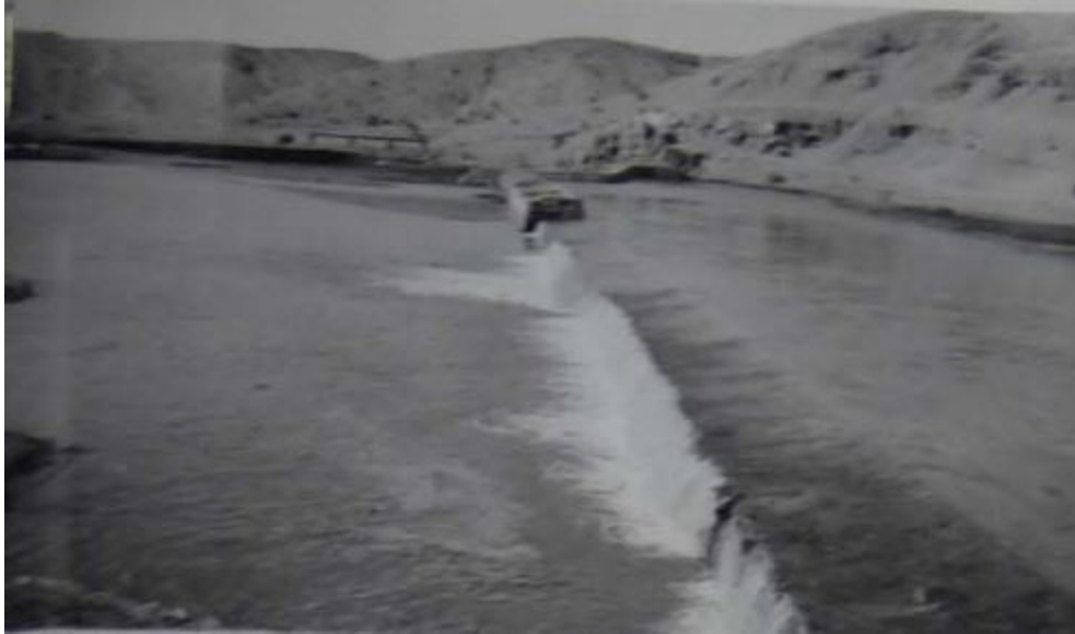
Head wall of Acequia Madre (foreground) with water recorder and bridge in background showing the absence of a control structure at the entrance to the canal - taken from the American end of the International Dam. Records of the Bureau of Reclamation. Engineering and Research Center Project Reports, 1910-1955, Box 722, Mexican Canal Diversions in the Vicinity of El Paso. U.S. National Archives, Denver.
