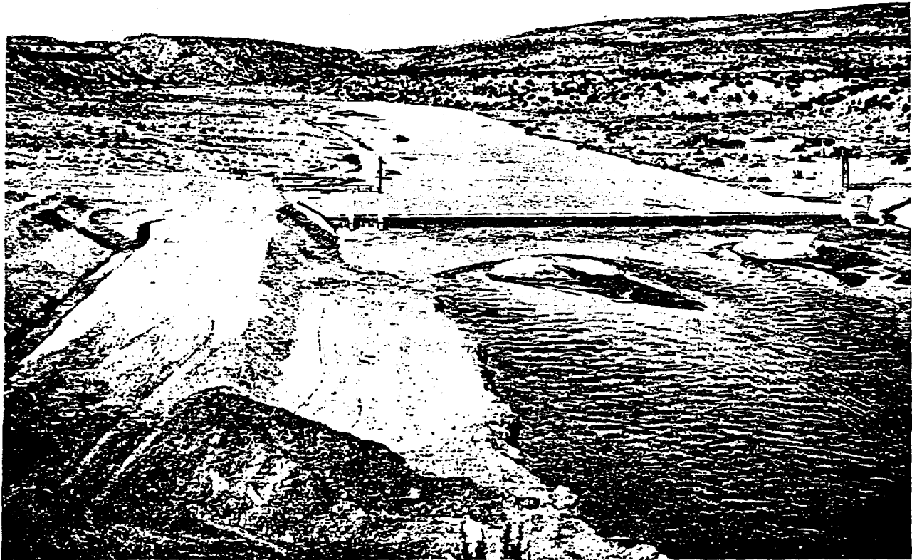
FIGURE 2—Cochiti Diversion Dam, Middle Rio Grande Conservancy District, New Mexico
